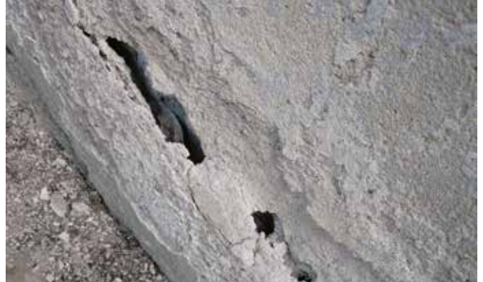
Damaged plaster
